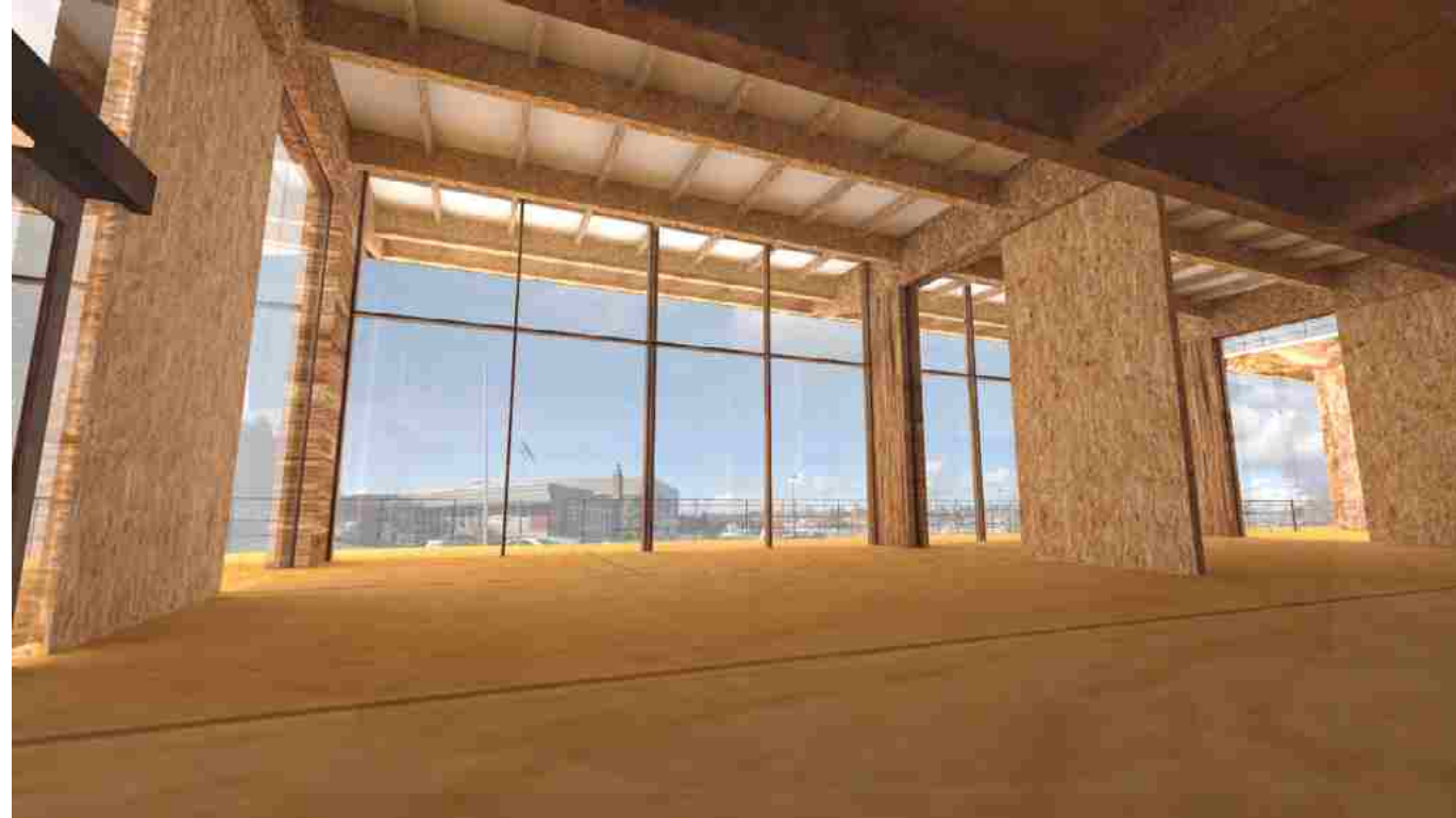
FIGURE 26: Interior rendering of 2nd Level space, looking west from under loft floor. Engineered wood systems serve dual purpose as finished interior surfaces, exposing the nature of the structural system. The building is insulated on the exterior of the structure below the cladding system. The raw interior expresses the intended programmatic uses of the interior, but allows for refinement and flexibility for any future changes in the program of the building.
